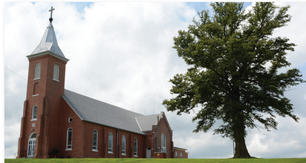
St. Anthony's Church near West Point is oldest parish in rural Omaha Archdiocese.
